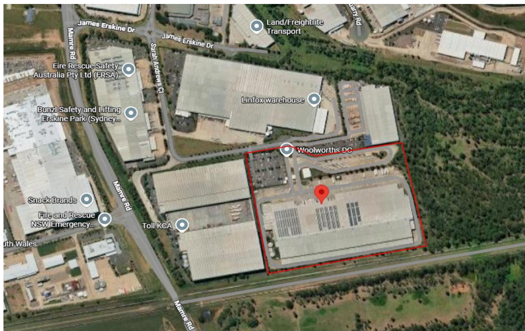
Figure 2 - EPDC Premises overview showing neighbouring properties
